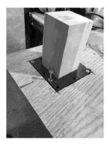
Tip: Ensure you know how each wood type will hinder or ease your installation. Also, ensure you check the level of your post after securing it as it may be angled slightly to one side. It is best to tip the post 1/2 of a degree inwards toward where the rail will be connecting to help keep everything in place over time
