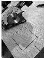
1. Trace the outside of your plate onto your subfloor and, using a skill saw, cut out a 6" x 6"x at least 1/4" deep square
