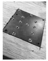
3. Ensure the base plate fits flush within the cutout, with enough space around the outisde to allow for small rotational corrections
