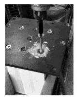
5. Screw your #10 wood screws into the holes to secure the plate to the bottom of the post
