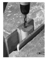
7. With a 3/8" drill bit, drill into the marked centre point from the end of the rail until the two holes intersect
