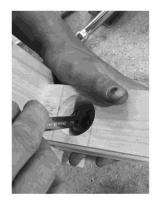
9. When satisified, apply wood glue to the end of the rail, and resecure the nut and washer, tightening as much as the wood type will allow. Wipe away excess wood glue
